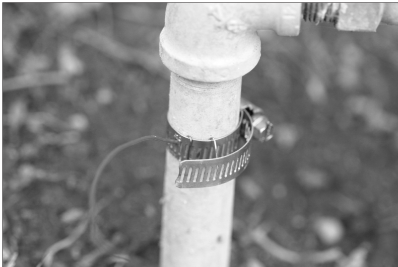
Figure 2-6: A good ground connection.
