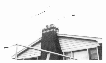
Fig. 13-6. JFD and RCA antennas mounted on the author's chimney, one above another. The upper antenna (RCA) supplies two outlets, while the larger (JFD) delivers good signals to four. No power is used, and 11 Washington-Baltimore stations are received, most of them very well.
