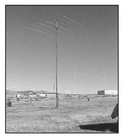
Fig 18—Installation of surplus AB-577 tower with tribander at 45 feet at K7NV. (*Photo by Kurt Andress, K7NV*.)
