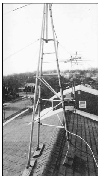
Fig 43—This tripod tower supports a rotary beam antenna. In addition to saving yard space, a roofmounted tower can be more economical than a groundmounted tower. A ground lead fastened to the lower part of the frame is for lightning protection. The rotator control cable and the coaxial line are dressed along two of the legs. (*Photo courtesy of Jane Wolfert.*)
