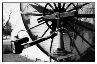
Fig 90—Elevation system, showing modified TVRO mount.
