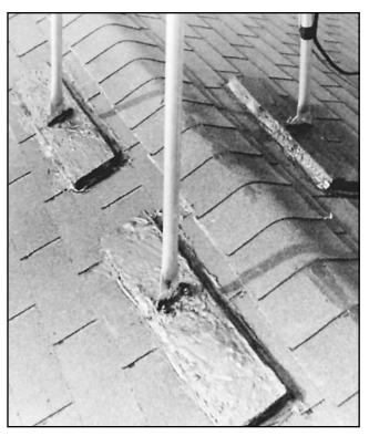
Fig 45—Three lengths of  $2 \times 6$  wood mounted on the outside of the roof and reinforced under the roof by three identical lengths provide a durable means for anchoring the tripod. A thick coat of roofing tar guards against weathering and leaks.
