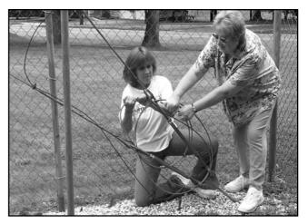
Fig 24—A length of guy cable is used to assure that the turnbuckles remain in place after they are tightened. This procedure is an absolute requirement in guyed tower systems. (*Photo by N4QX*)
